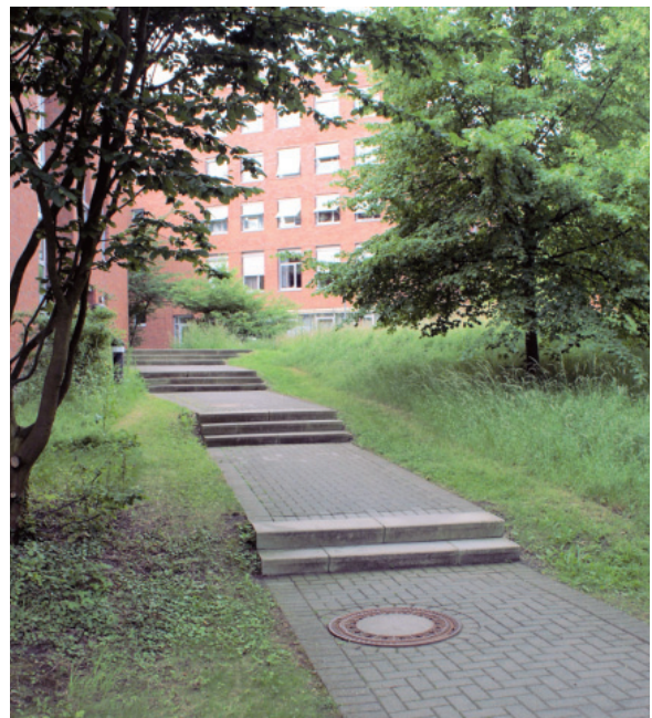
Picture 3 Slopes causing problems for mobility impaired people or wheelchair
